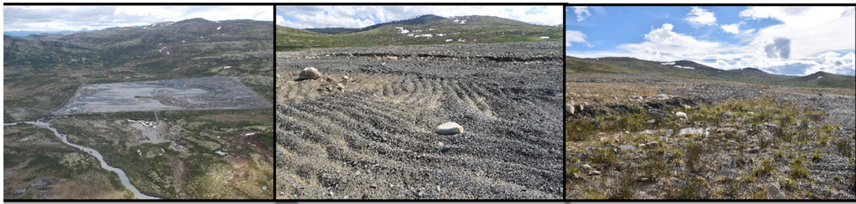
Fig. 4. a) Restoration of a 600 × 400 m large homogenous testing field included land shaping in 2013, b) tilling of surface soil in 2013, c) seeding of native Festuca ovina and planting of local willow-species ( Salix glauca , S. lapponum and S. phylicifolia ) in 2014 to improve conditions for long term vegetation recovery, as observed in 2020.
