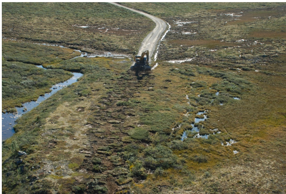
Fig. 3. Standard method to remove roads included removing added gravel, reshaping original terrain surface and transplanting turfs from road verges to wipe out the artificial borders and promote vegetation recovery.
