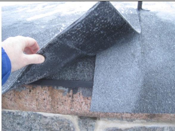
19.1.2011 Overlapp over gammel kantavslutningslist.
