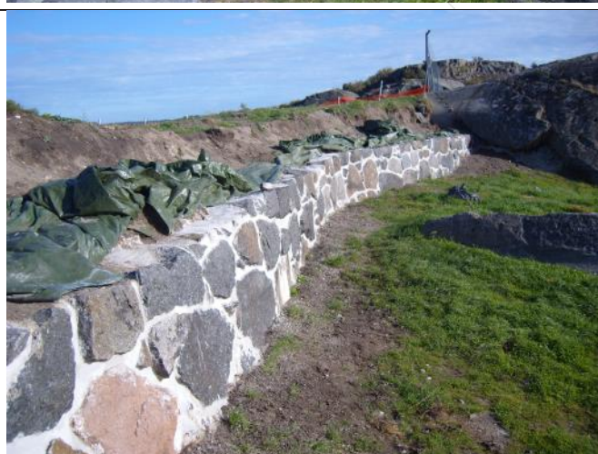
Ferdig mur innside
